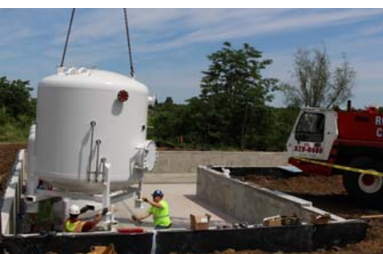
Granular activated carbon tanks being delivered and installed.
